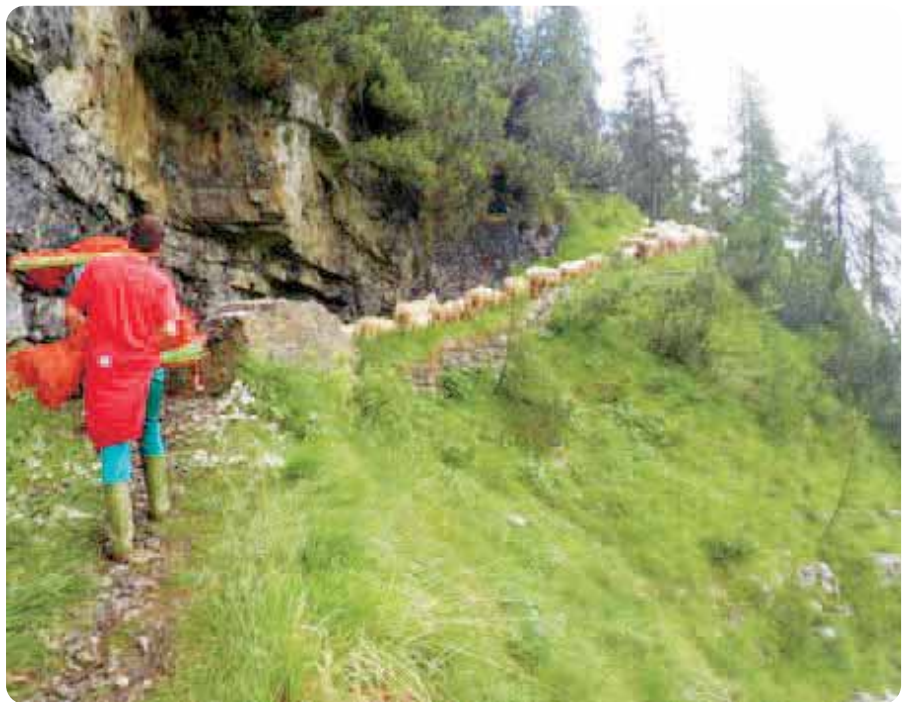
Photo 9 - Transport of electric fencing to location at high altitude
